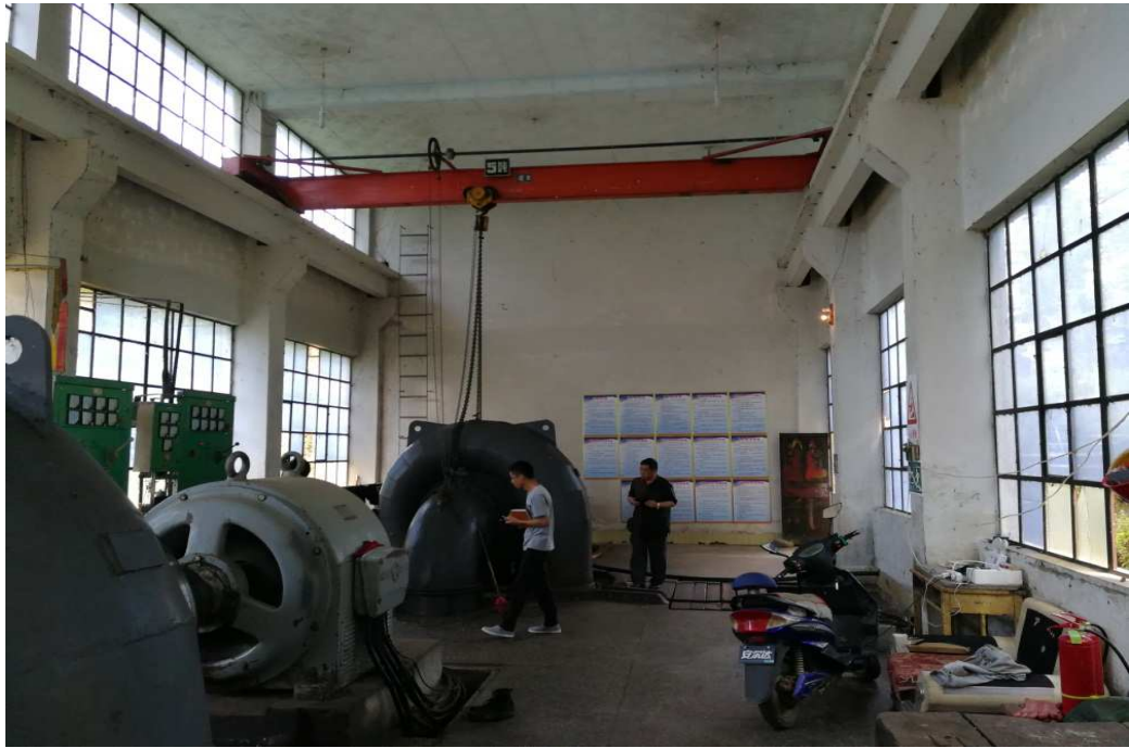
盐井电站厂房踏勘
