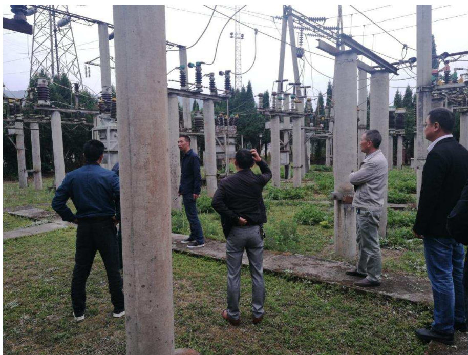
观音岩电站升压站踏勘
